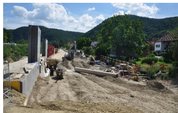
Figure 10: Flood protection under construction along the Danube in Rossatzbach (2022) (C: Department of Hydraulic Engineering WA3)
