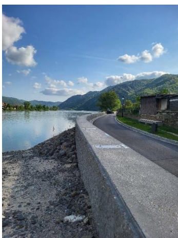
Figure 9: Completed flood protection along the Danube in Bacharnsdorf and Mitterarnsdorf (2024) (C: Department of Hydraulic Engineering WA3)
