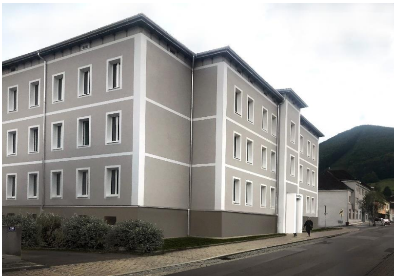
Figure 4: Refurbished office building 2 Lilienfeld, (Source: LAD3)
